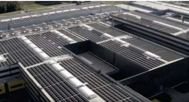
COMPACTFLAT, 6,9 MW, Austria
