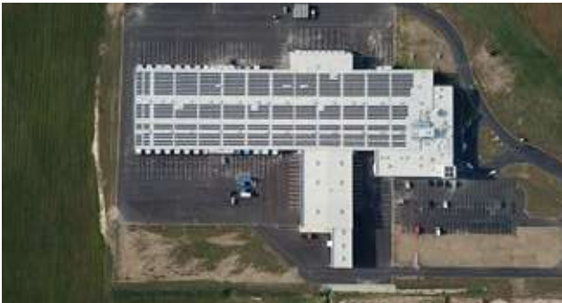
COMPACTFLAT, 500 KW, Estonia
