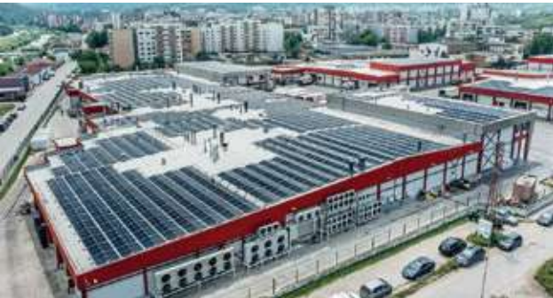
COMPACTFLAT, 1,779 kWp, Bulgaria
