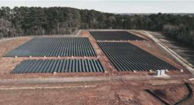
COMPACTGROUND, 1,3 MW, USA
